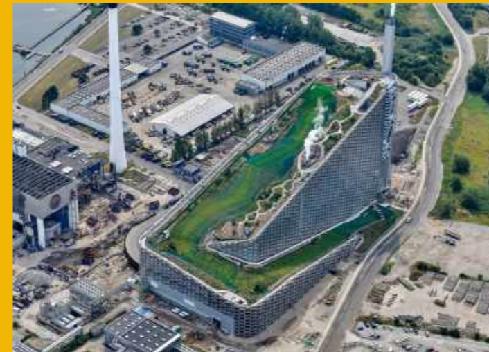
‘Waste-to-energy’ plant, CopenHill in Denmark, featuring a ski slope and hiking trails Credit: istock
